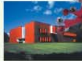
The Regional Foundation for Contemporary Art in Carquefou
